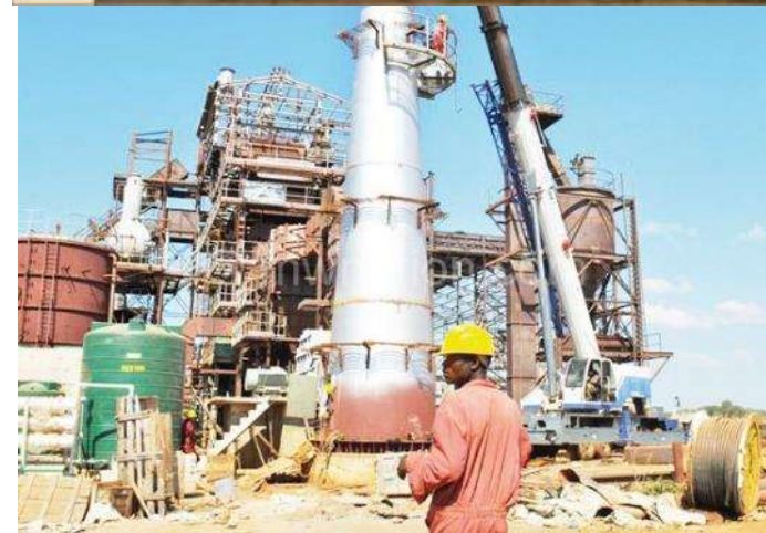
Under construction: The Chikwawa Green Belt Initiative sugar mill
